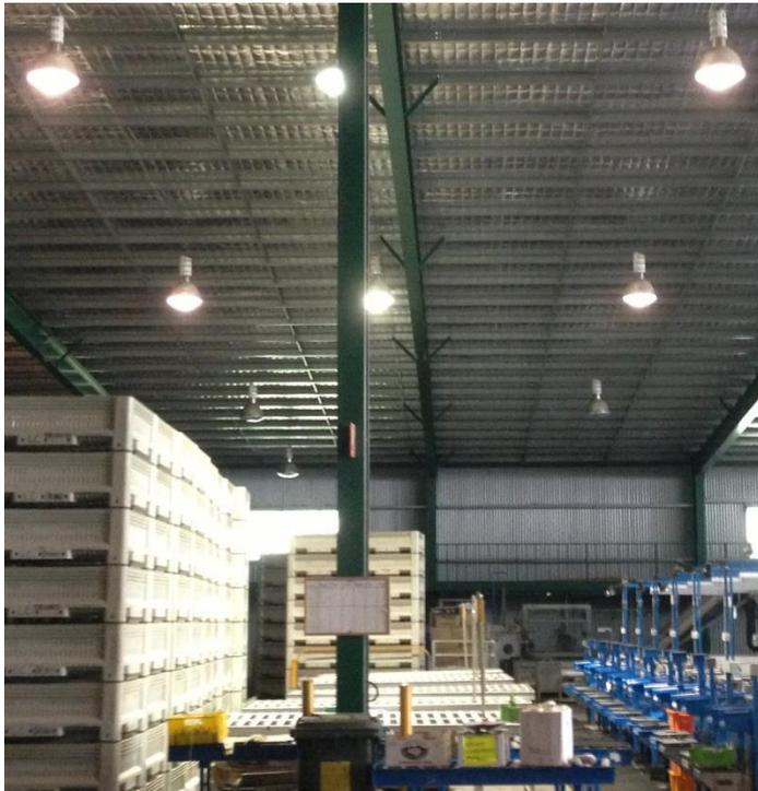
Metal Halide lights are often used in high ceiling spaces of packhouses and can be replaced with LED highbay lights that last a lot longer.
