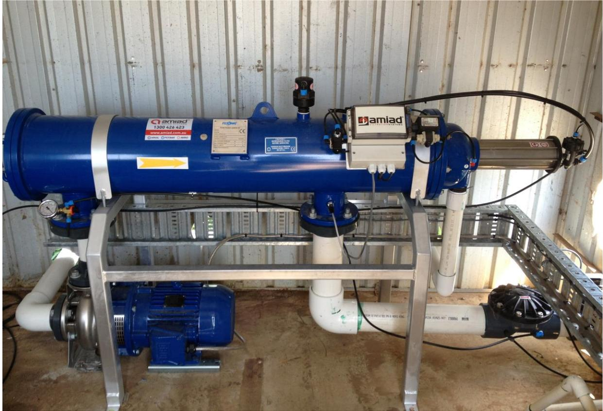
*A pumping station with a high efficiency motor connected to a variable speed drive that is automatically controlled. FS2 (Sep 2014)*
