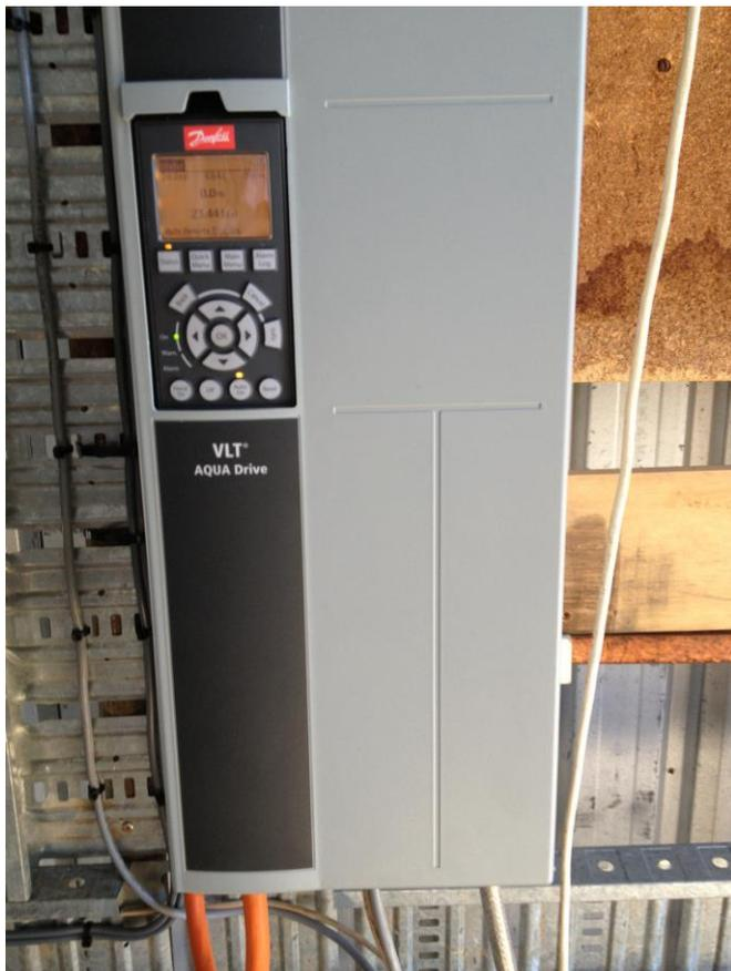
*A variable speed drive connected to an irrigation pump regulates the frequency of the electrical power supplied to reduce energy use.*
