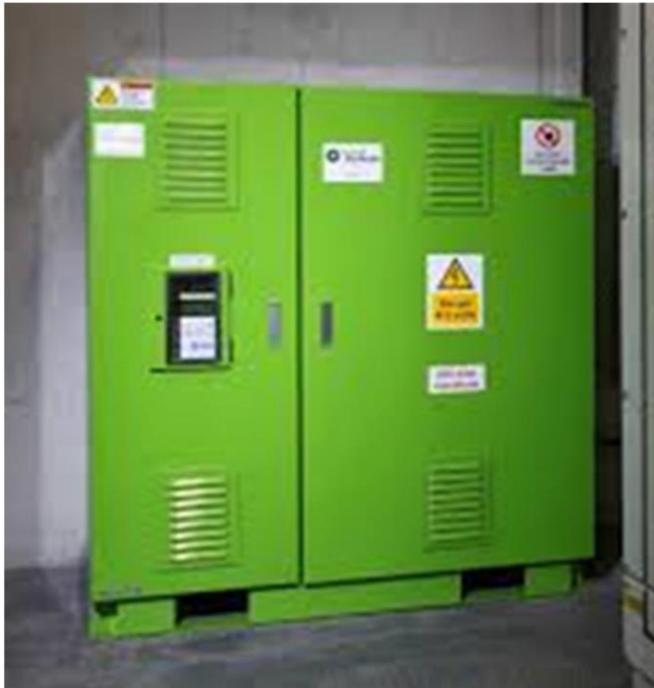
***A Voltage Power Optimisation unit can be installed on the building's main electrical supply to reduce electricity costs.***
