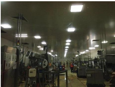
***Figure 3: Metal halide low bay light fixtures in Capilano's packaging area***
