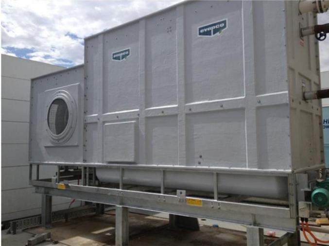
Radevski's have installed Evapco condensers at the Benalla Rd plant that use variable speed drive-controlled fans to reduce energy use.
